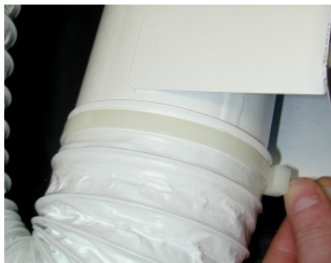
5) Fit new strip, tighten and cut over.
